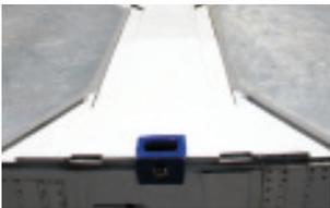
Casting extended into stacking lift post to provide over-lapping "hinge-free" weld joints for a stronger joint connection
